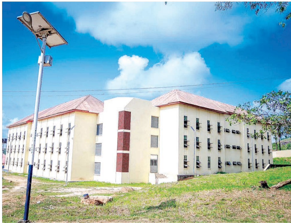
Renovated hostel at the Abia State University.
